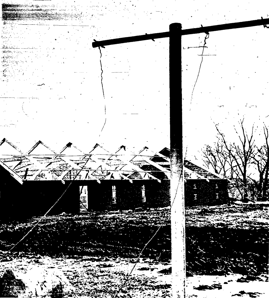
TRINITY LUTHERAN CHURCH at Hoskins is erecting this new sanctuary and educational unit at a cost slightly less than $100,000. Beams were installed Wednesday and
